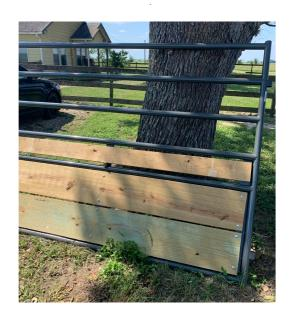
**Flush Fit** Picture Below Shown With 2" x 8" Board with 1/4" or so Ripped of edge to Fit "Varies on Lumber"
