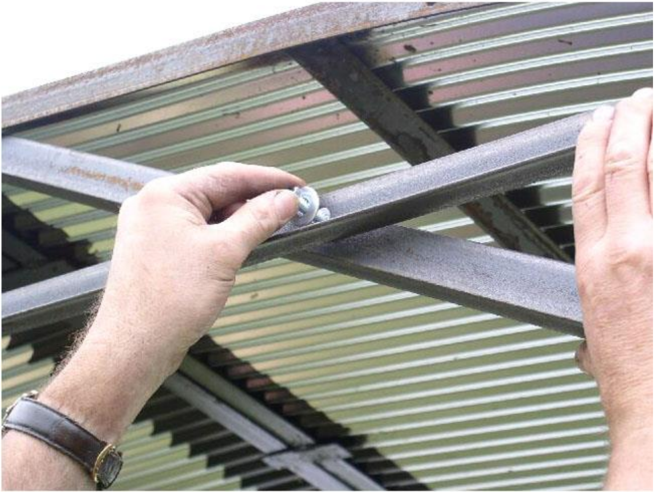
11. Bolt the braces together.
